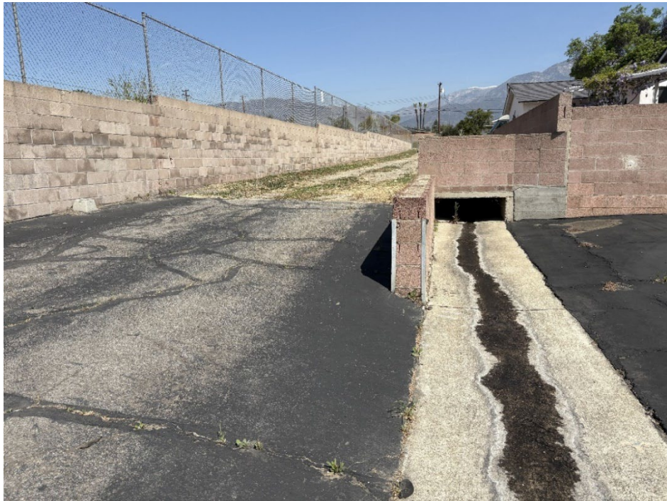
Photo 19: Culvert on eastern edge of BSA.
